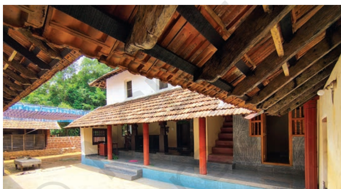
Figure 3.3: A traditional south Indian house with wood used for building roofs, doors, windows and pillars
