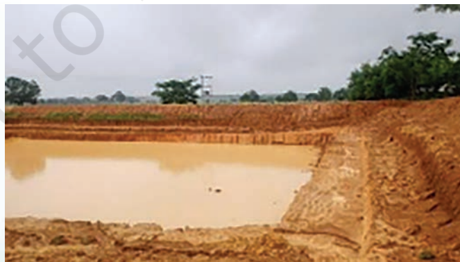
Figure 5.13: Percolation tank for groundwater recharge
