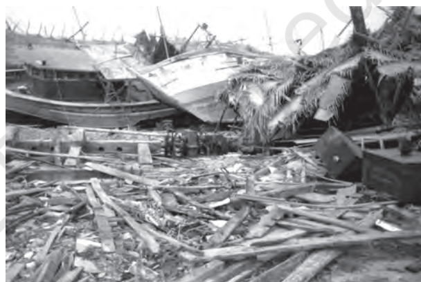
Figure 6.3 : Tsunami Affected Area
